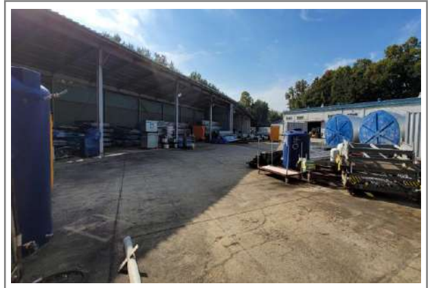
▲ Outside the factory building
