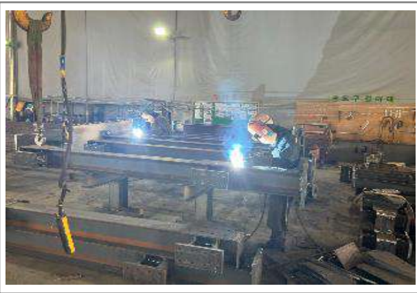
▲ Pipe Rack Production
